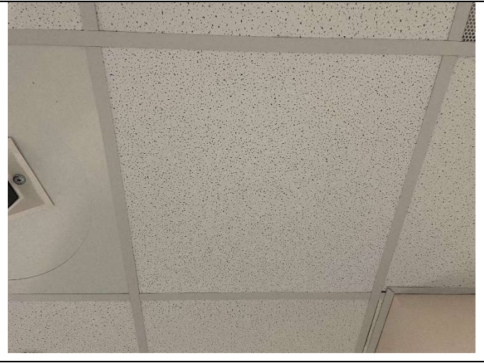
Photo 4: HM-C: 2' x 2' Ceiling Tile, White Pinhole
